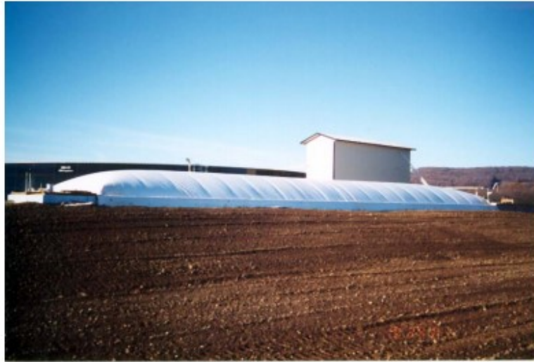
Figure 2-6 A dairy farm anaerobic digestion system\
