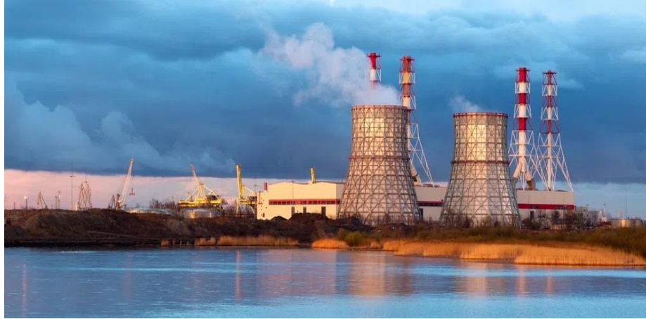
Fig.10.7: The two wide, concave structures are cooling towers.
