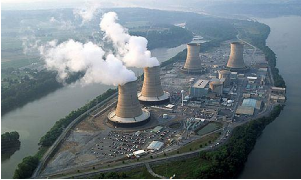
Fig.10.2: Wastes Generated at Nuclear Power Plants
