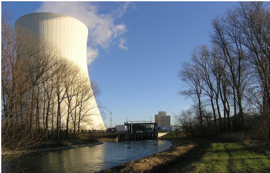
Fig.10.5: Cooling tower and water discharge of a nuclear power plant
